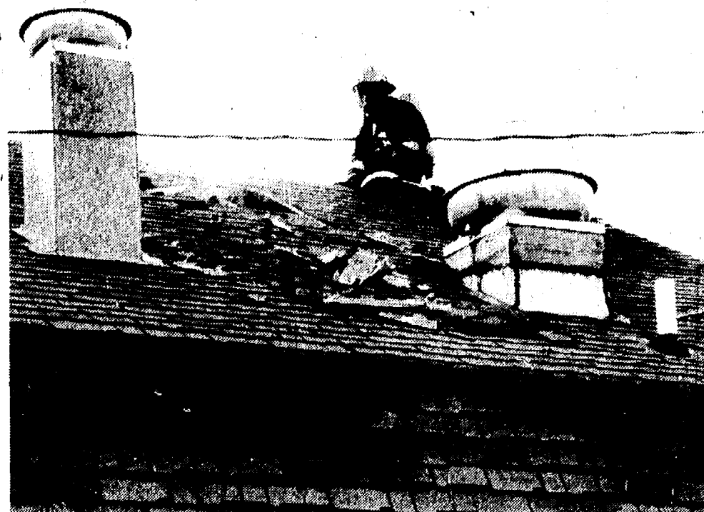
A VENT was cut in the roof of Lee's Hoagies as firefighters worked to contain a blaze at the restaurant Monday morning. The vent allows heat and smoke to escape. Excess heat can sometimes cause an explosion.
